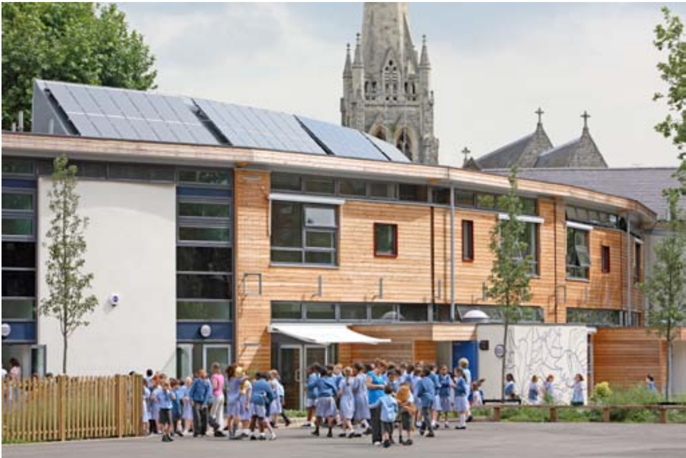
Solarcentury installation at Larmenier School, Hammersmith, London
