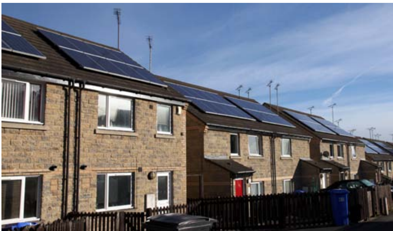
SYHA's 'Power Roofs' programme
